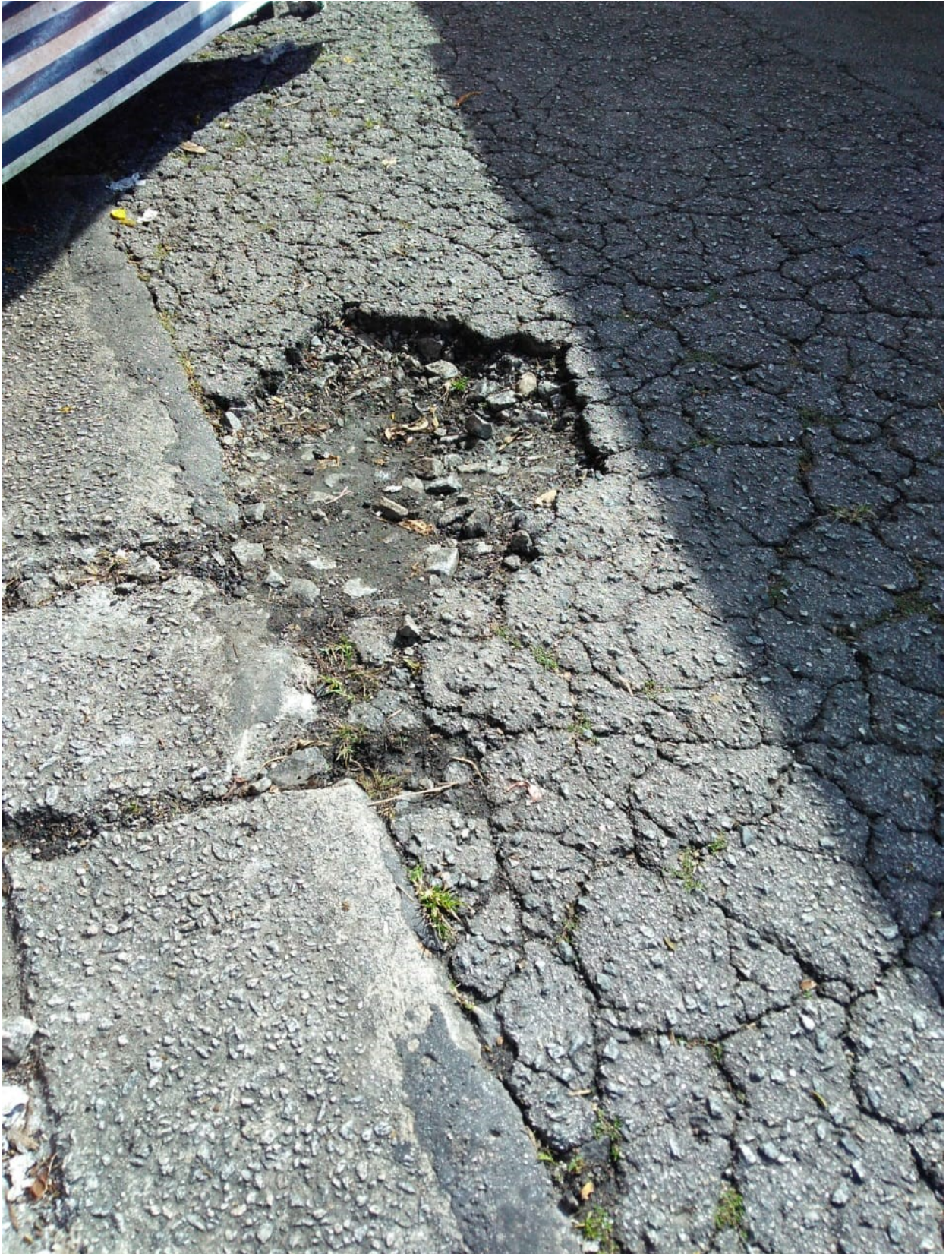
Rua Bauru – Tapar Buracos
